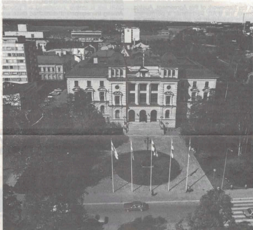
View of Oulu City Hall
